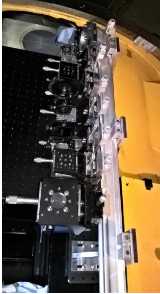
Figure 1. Shack-Hartmann wavefront sensor installed at THEMIS telescope.
